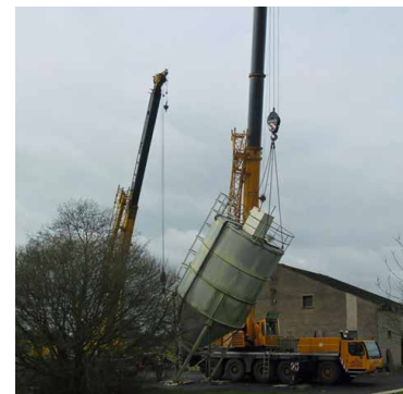
Silo Installation (Tandem Lift)
