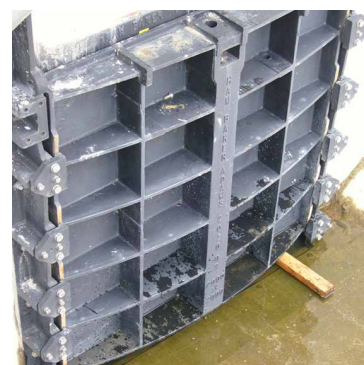
Refurbished Penstock Gate
