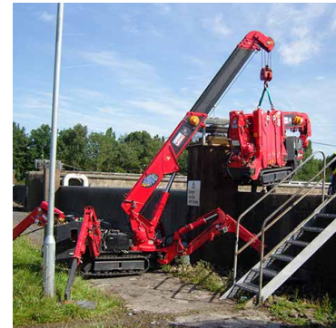
Spider Crane Lifting a Spider Crane
