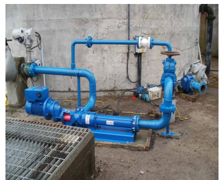
Pump and Pipework Replacement
