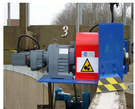
Tank Drive Upgrade
