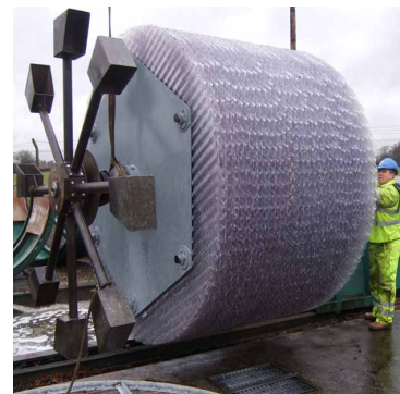
RBC - Repairs and New
