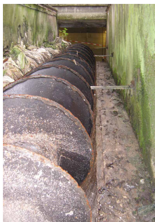
Worn Archimedes Screw
