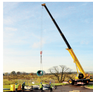
On-site Crane Lifts
