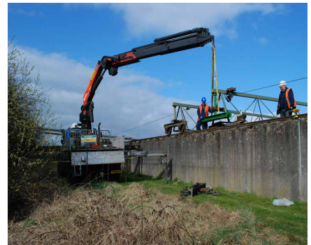
Bridge Carriage Replacement
