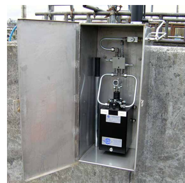
Manually Operated Hydraulic Pump
