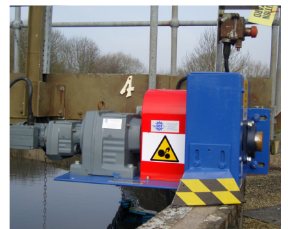
Tank Drive Replacement
